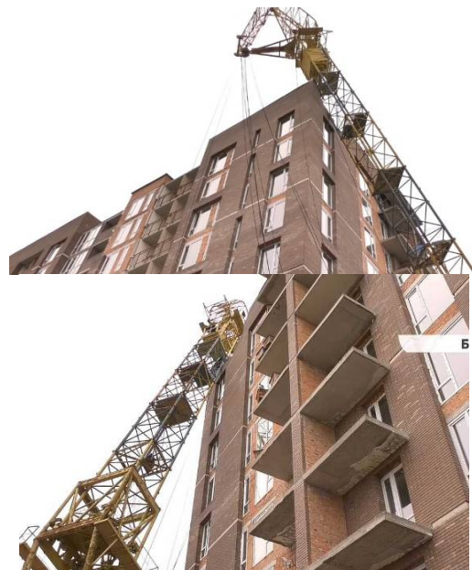
Fig. 6. The fall of the tower crane KB405.1A in the city of Bucha
