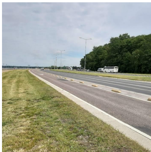
Figure 7: plastic "armadillos" on the Pirita Highway, Tallinn, Estonia. The photo by Anton Klymenko.
