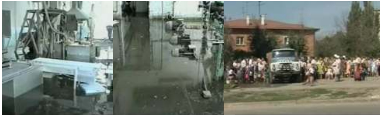
Figure 3.3 - Consequences of the accident at the Dykaniska pumping station, 1995
