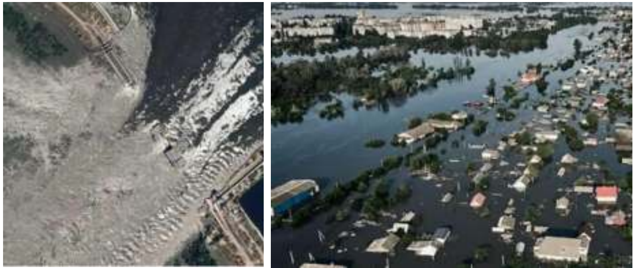
Figure 3.2 - Consequences of the destruction of Kakhovka HPP
