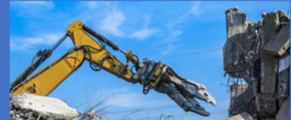
Dismantling of of destroyed facilities
