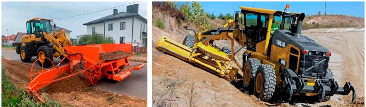
Figure 1 – Work during laying and widening of road shoulders
